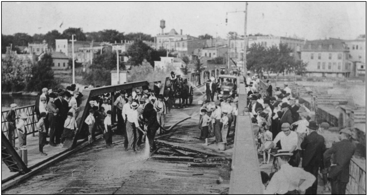
A crowd gathers to watch work on the wooden planking of the bridge deck in the early 20 th century.
