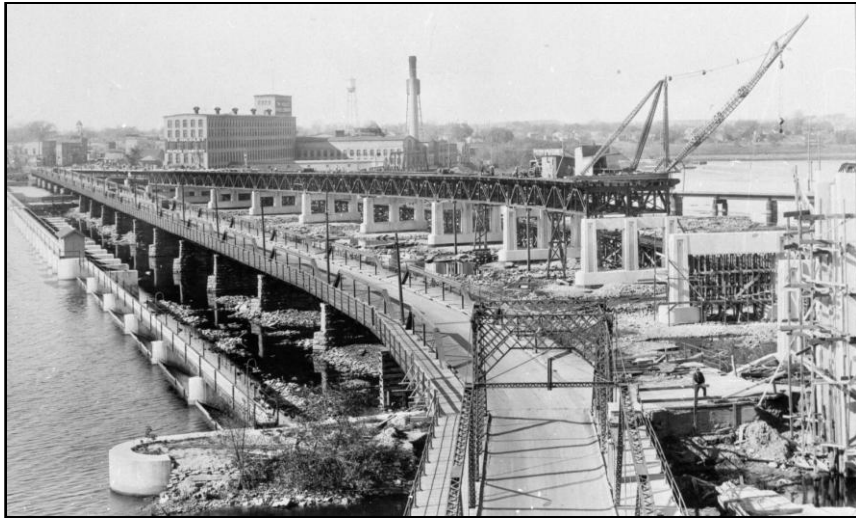
Construction of the Claude Allouez bridge in 1932.
