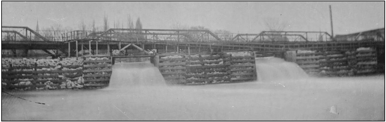
Crib dams were wooden structures filled with rocks. The force of the water as it rushed through the sluice or openings between the cribs created the waterpower used by the mills along the river.
